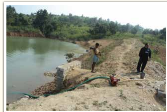
Construction of Check Dam – Visit by Late. Father Ranjeet
