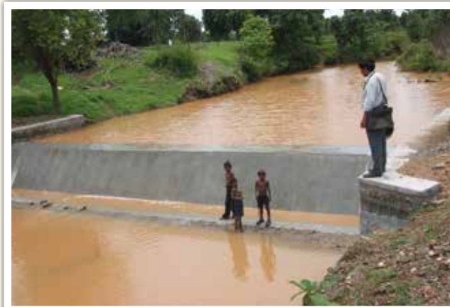
Check dam at Hindalco Muri
