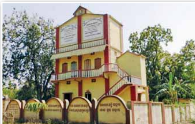
Water Tower for Supply of Water at Lakhanpur, Odisha
