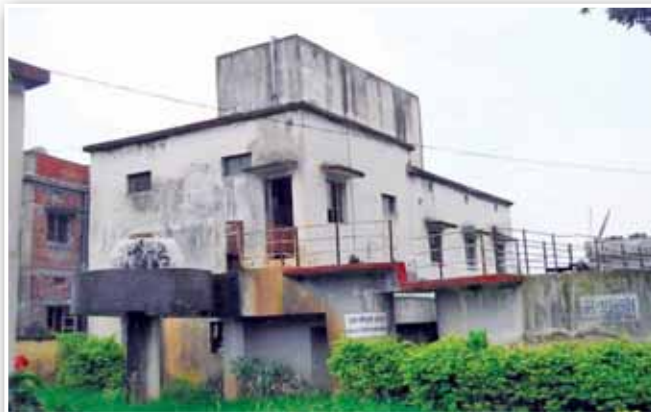
Water Treatment Plant at Khijri, Jharkhand
