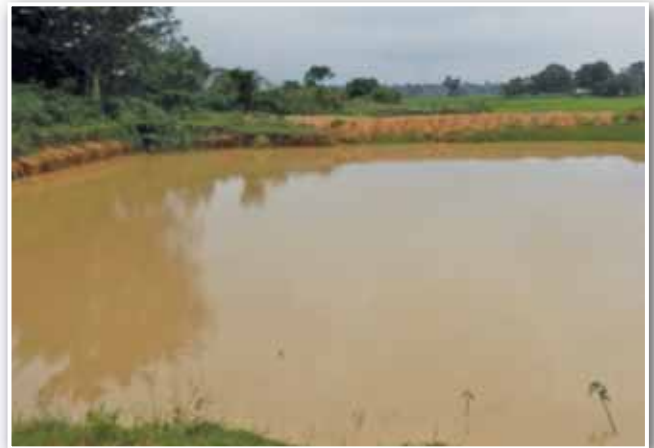
Check Dam constructed for irrigation
